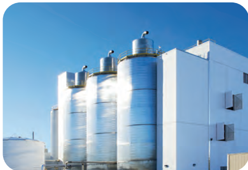
THE WORLD'S LARGEST BIO-BASED SUCCINIC ACID PLANT, SARNIA, ONTARIO.
